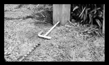
The gap between the centre of the top gudgeon hole and the centre of the bottom gudgeon hole should match exactly the distance between the hinges on the gate. Drill this hole on the same angle as the top gudgeon (positioning the gudgeon on the ground as a guide may help). Again, check that the drill bit is horizontally level before you start drilling. Insert the gudgeon, mark and drill the hole for the locking tail. Insert the locking tail and hand-tighten the gudgeon's outer nut.
