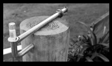
When mounting gates to timber strainers it's best to use Through Post Gudgeons, which go all the way through the strainer for extra strength and adjustability. Greyson or Franklin Lock Thru Post Gudgeons (with a hook-like 'locking tail' under the pin) are a good choice as they won't twist in the strainer. Each gudgeon needs to be long enough to easily pass through the centre of the strainer, comfortably allowing enough excess to attach and adjust the outer nut.
